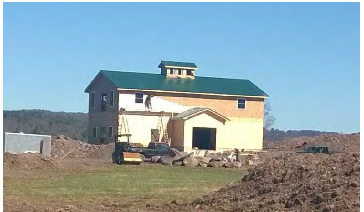
The new Handsome Brook Farm barn on Franklin Heights
