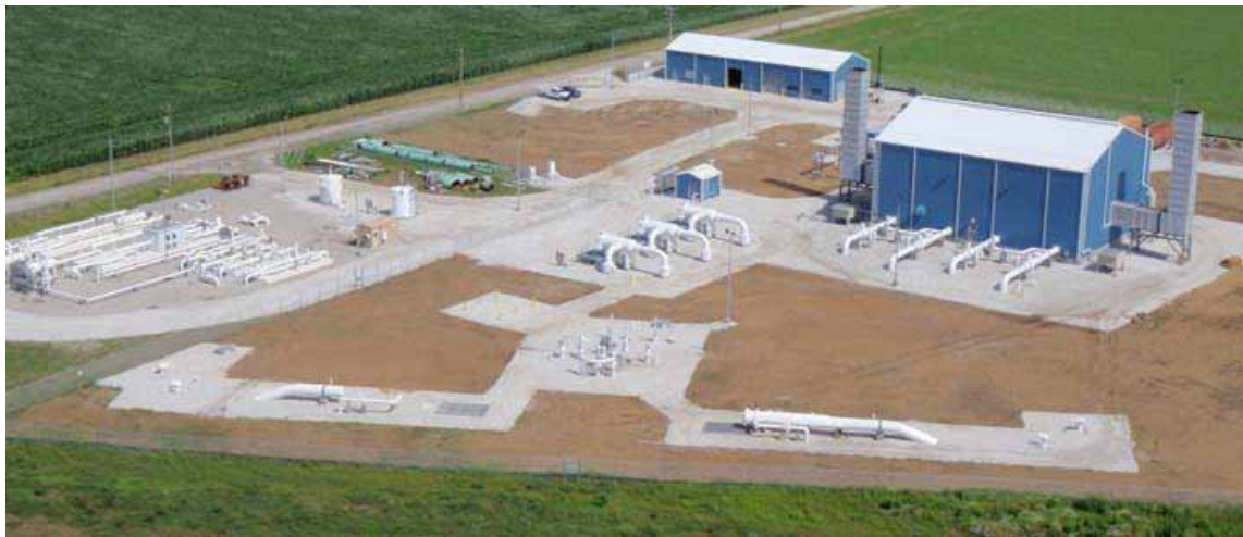
Kinder Morgan’s Mexico compressor station on the Rockies Express pipeline. Two Titan 130 turbines are housed in large building, upper right. Photo: Alliance Wood Group Engineering, L.P
