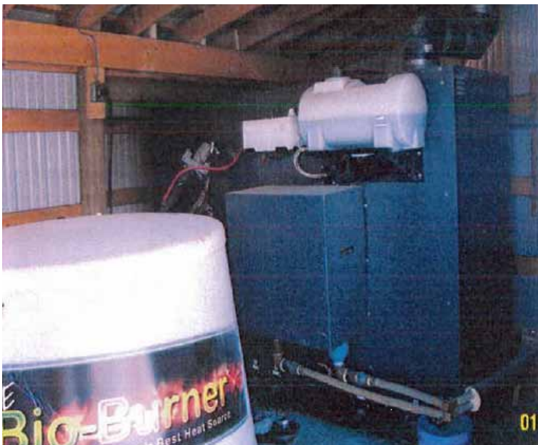
The second grass pellet boiler at the Franklin town garage in a shed built for it by the town. The water tank above the boiler is part of the fire-suppression system.
