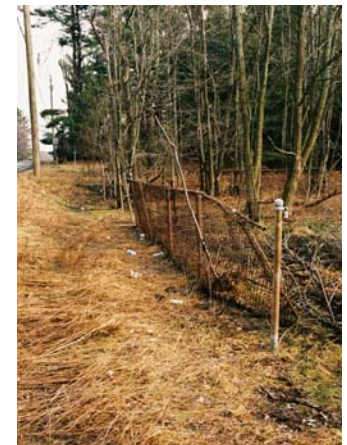
Chain link fence in disrepair
