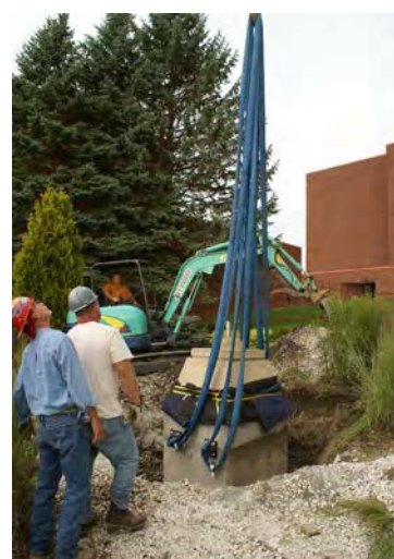
Harp base is attached to crane
