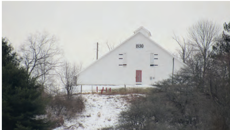
Reservoir building seen from Otego Mountain Rd. Photo by author
