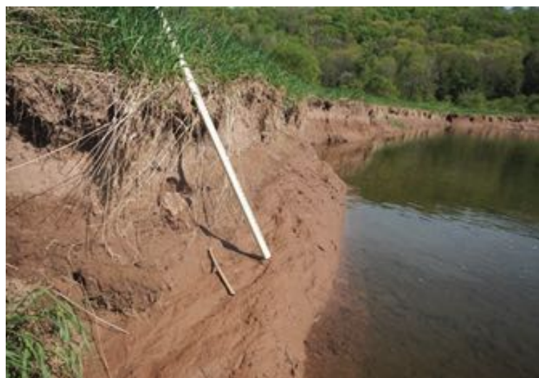
Streambank erosion along the Ouleout Creek Photo: DCSWCD
