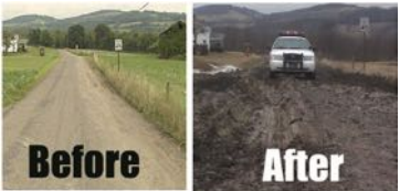
Typical road damage from heavy use
