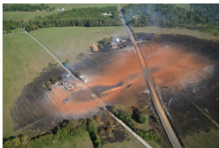
Photos of the September 14, 2008 Williams Transco Pipeline explosion in Appomattox, Virginia.
