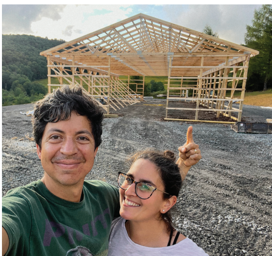
Pole barn construction begins!
